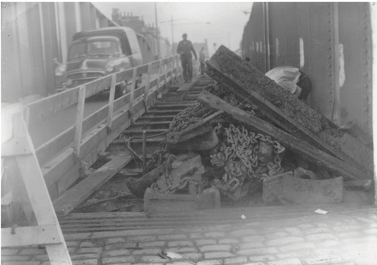
Old ballast being removed during refurbishment of the bridge in June 1960.
