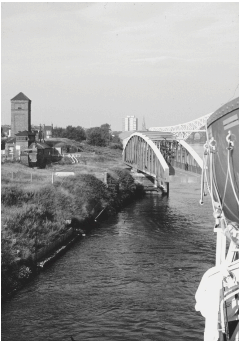
The Old Quay Bridge over the Manchester Ship Canal at Runcorn. The tower for the hydraulic accumulator and the pump house are on the left.
