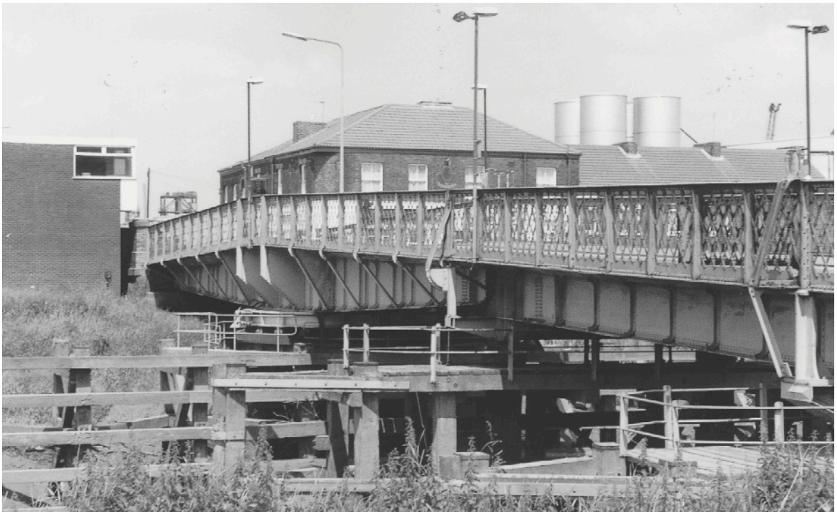
The swing bridge over the Dutch River at Goole.
