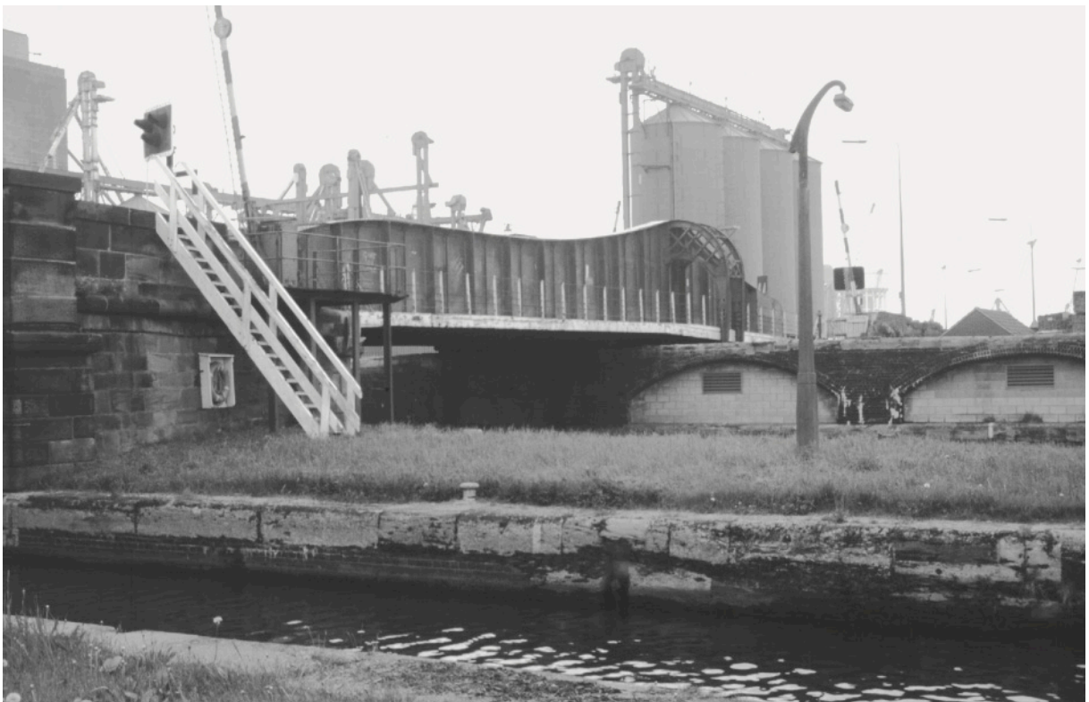
South Dock Bridge seen from the south east across the passageway opened in 1910. The bridge swings over the two arches, the operating mechanism being on the north western side of the bridge.
