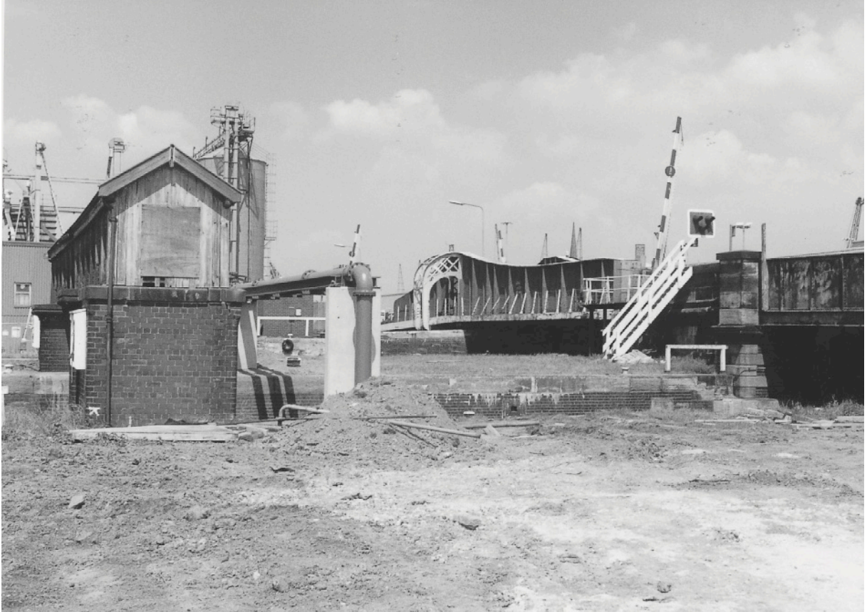
View of South Dock Bridge from the south west, looking across the passageway opened in 1910. On the right is the fixed plate-girder bridge over the passageway.
