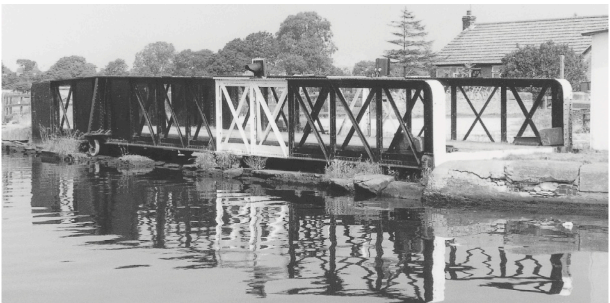
No. 3 Swing Bridge, situated just below Pollington Lock. This type of open lattice girder swing bridge was originally proposed for South Dock Bridge in the 1880s.
