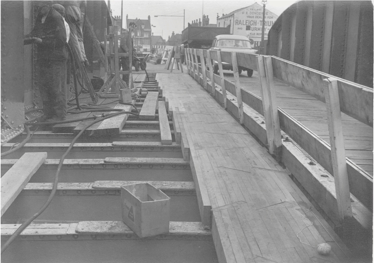
The replacement vertical planking during installation.
