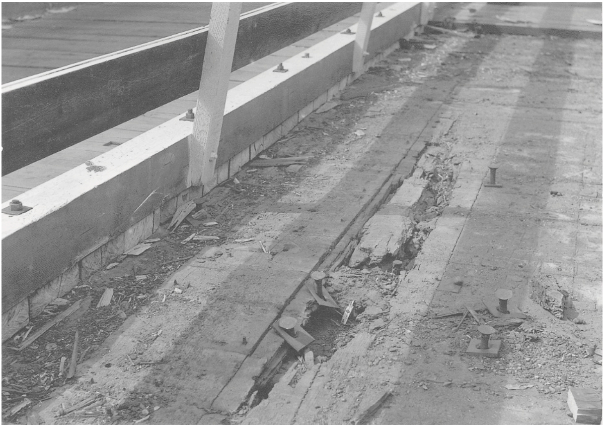
The old flat wooden deck planking pictured before replacement in June 1960.
