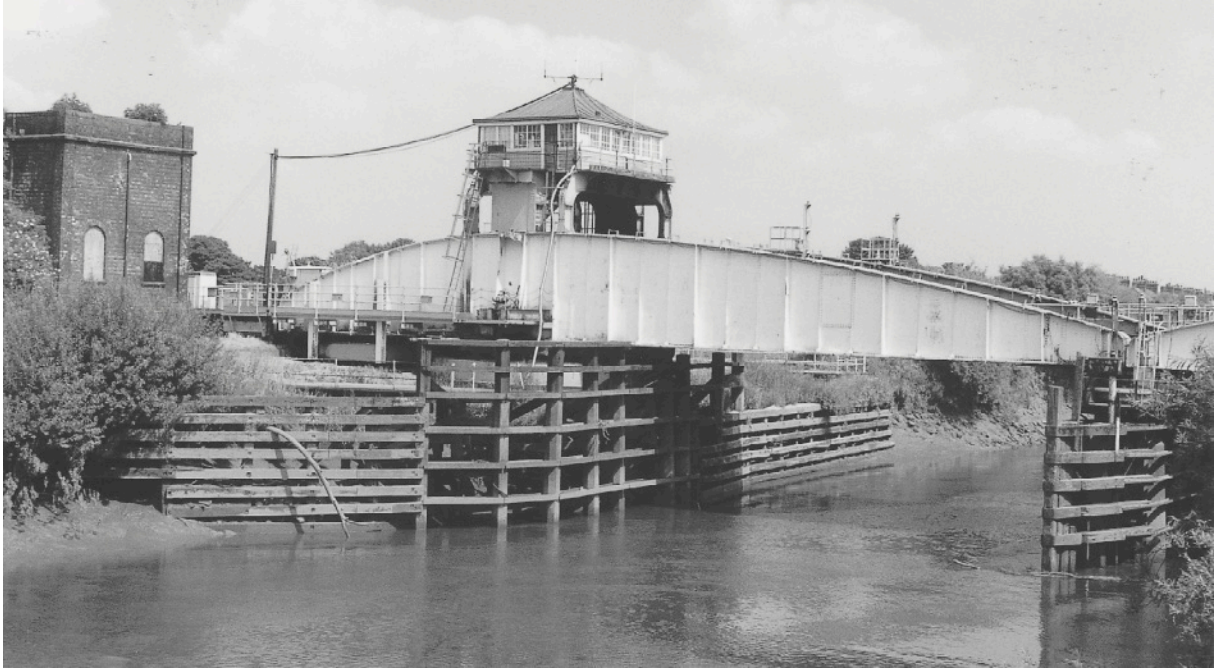
The railway swing bridge over the Ouse at Selby.
